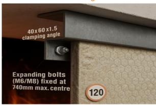
Attach 40×60×1.5 mm or 50×50×1.5 mm clamping angle with M6 expanding bolts at 740 mm centres. Use 5 mm bolts & nuts at 400 mm centres to secure blanket
